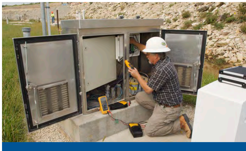
Bob Frazey works in one of the sensor service panels that lay across the base of the dam. These service panels are all low voltage panels that house ground swell sensor communications and support systems. He uses the Fluke 189 DMM to check the 12 V dc battery charging system that comes from a nearby solar panel. He also uses the Fluke 771 Milliamp Process Clamp Meter to check the 4 mA to 20 mA signal from the pressure sensors and transducers.
