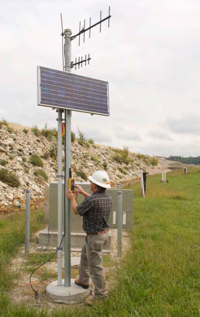
The Fluke 1630 is also used to check the grounding wire on the mast of the radio antenna and solar charging panel. Frazey also uses the Fluke 189 DMM with a Fluke i410 current clamp to look at the current output of the solar panel to the battery charger inside the service panel.
